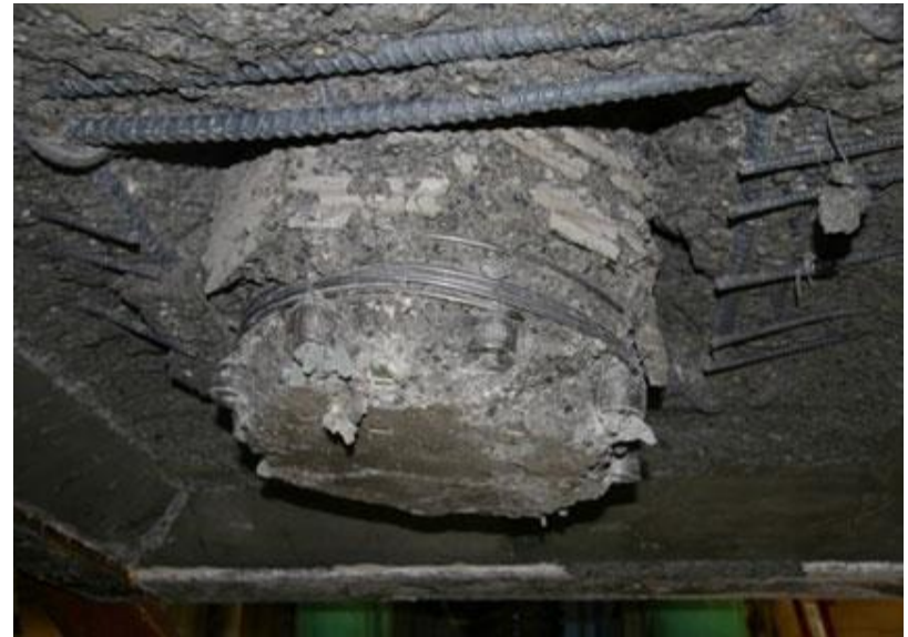
Location of critical shear section and perimeter
