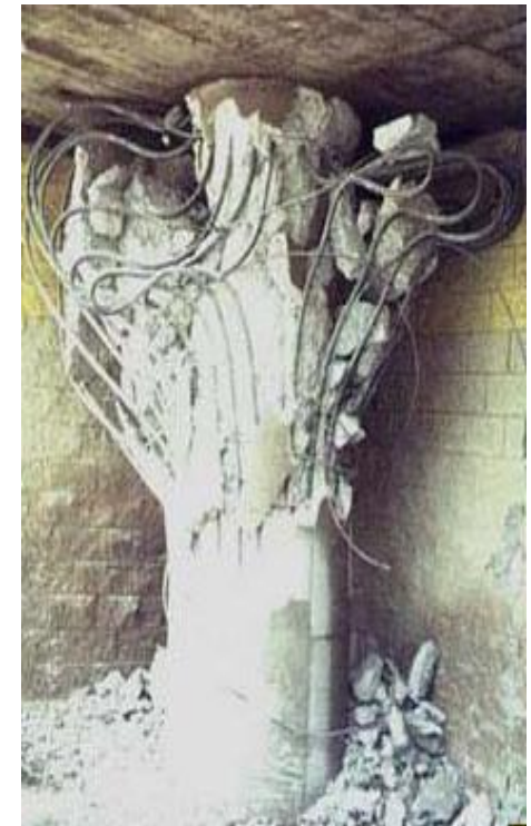
← Shear failure of a column of the Shinkansen bridge
