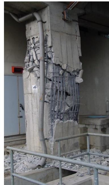
← Shear failure of a column of the Shinkansen bridge
