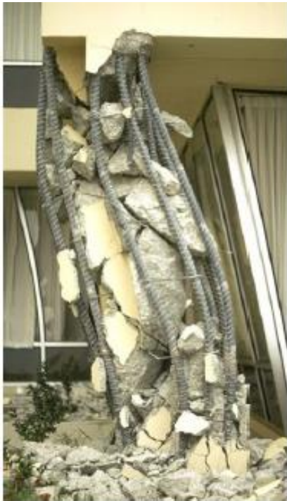
↑ Damage of circular column during earthquake due to poor detailing of transverse reinforcement
