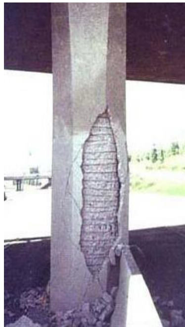
↑ Damage of circular column during earthquake due to poor detailing of transverse reinforcement
